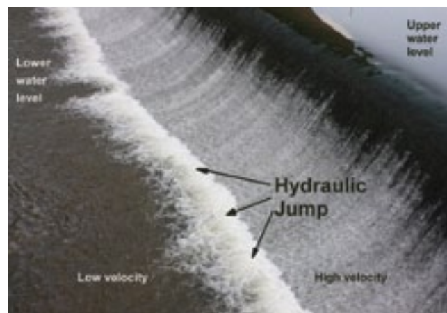
Figure 1: Hydraulic Jump at spillway
